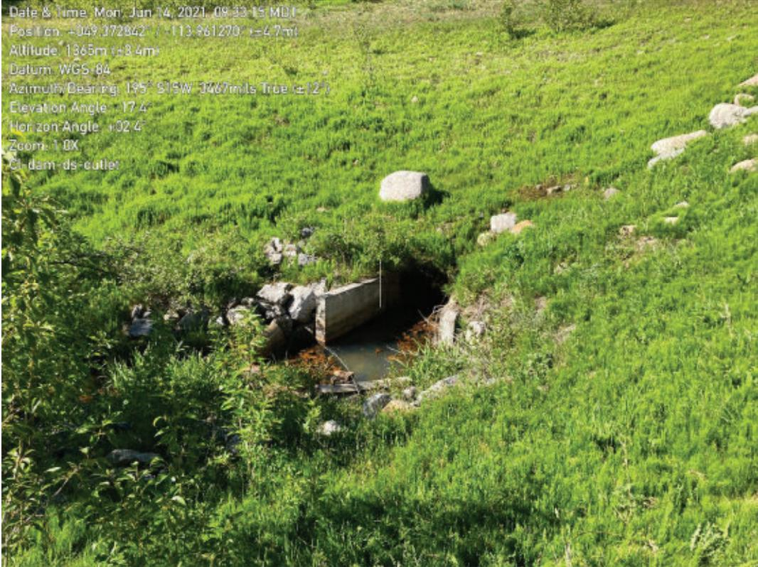
Photograph 1-15 Downstream outlet headwall at toe
