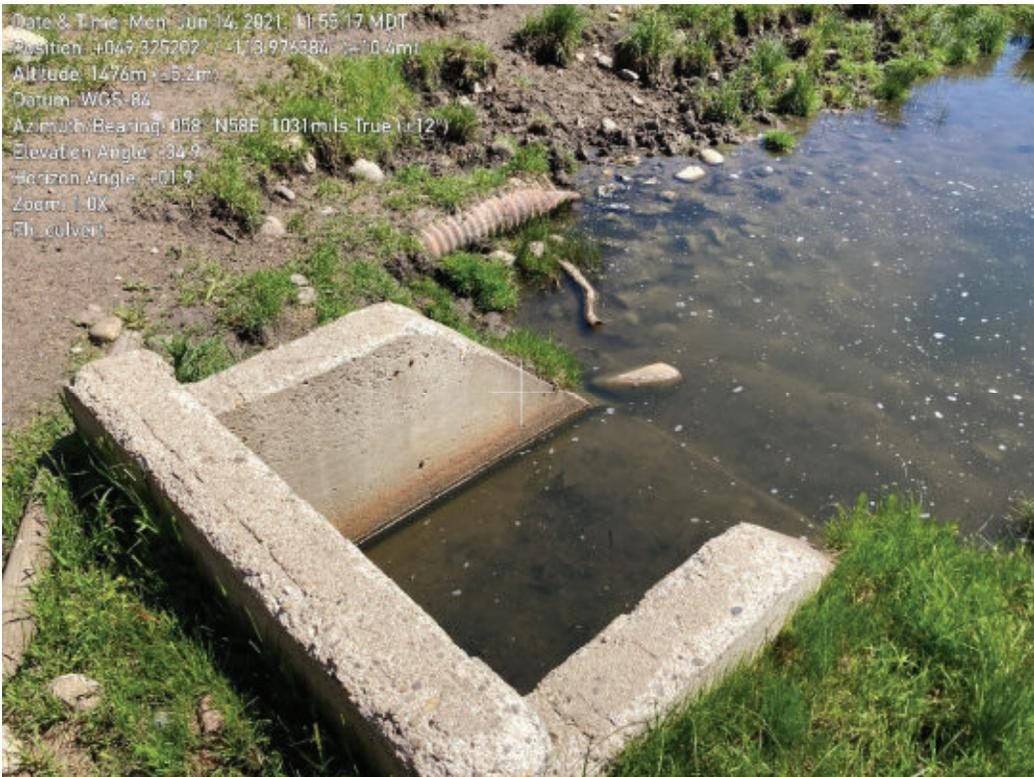
Photograph 5-12 Damaged CSP outlet culvert pipe head and headworks of low level outlet
