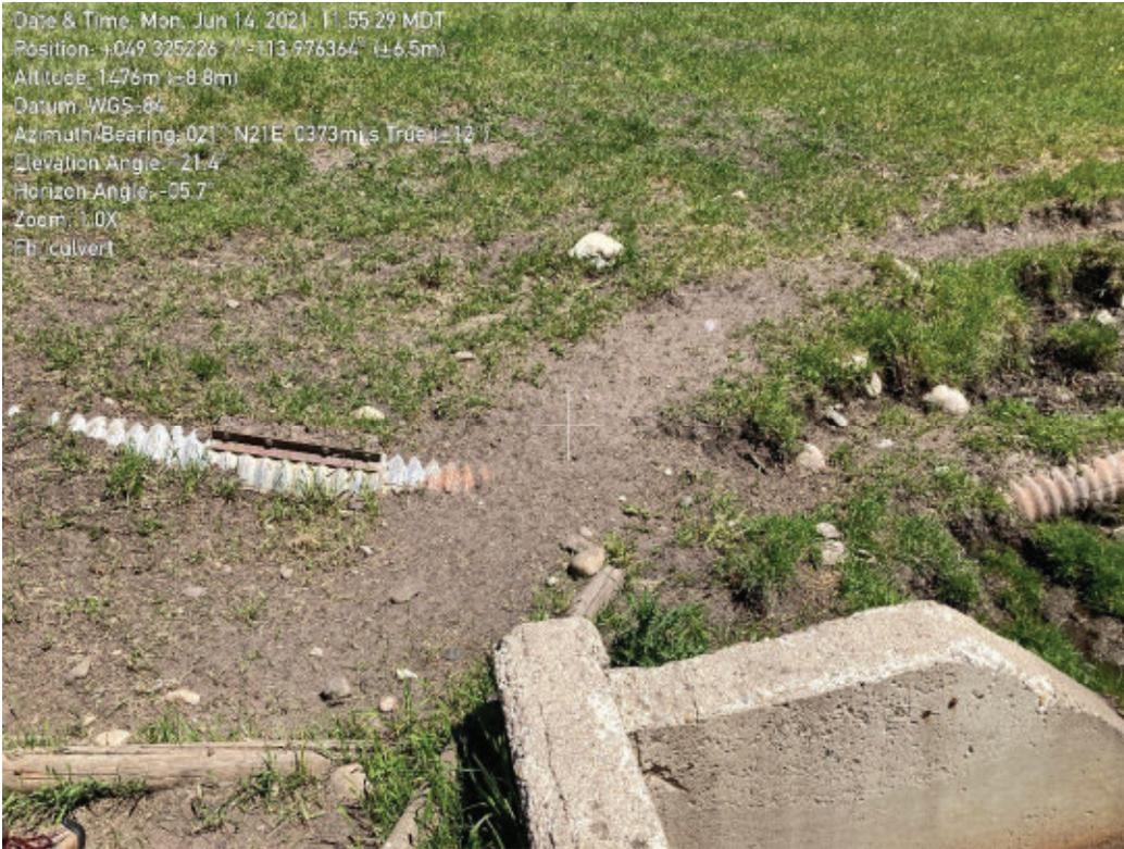
Photograph 5-11 Exposed CSP outlet culvert
