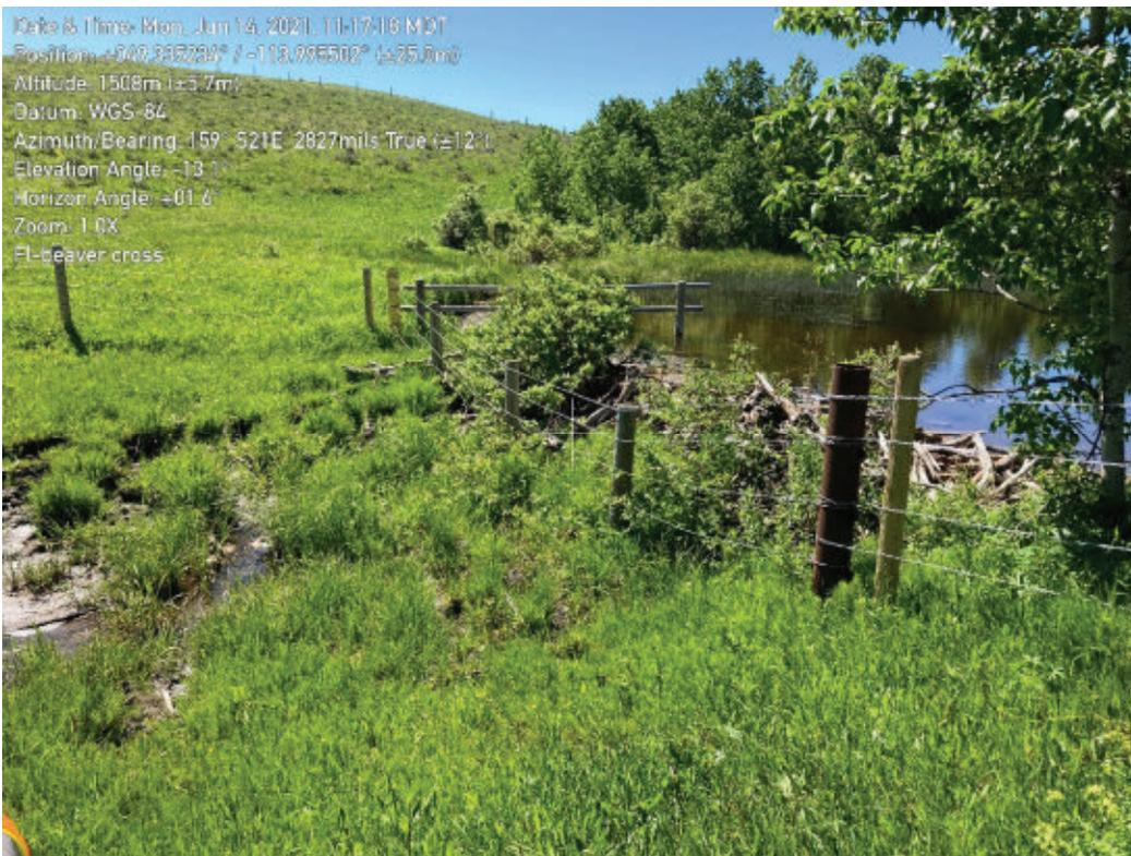
Photograph 4-6 Spillway channel blocked by beaver dam, facing south
