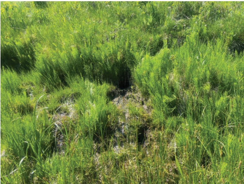
Photograph 2-16 Seepage and Standing water observed on downstream slope (natural section)
