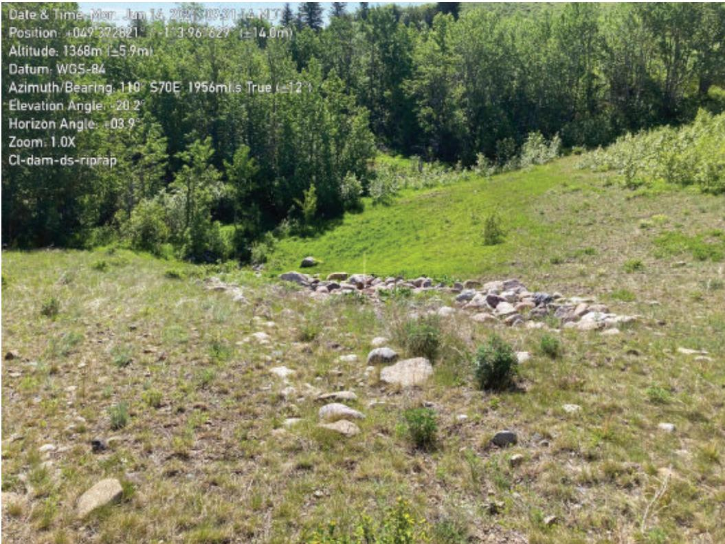
Photograph 1-10 Riprap on dam downstream slope – facing down
