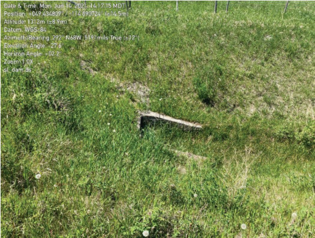
Photograph 3-3 Dam downstream slope and outlet headwall
