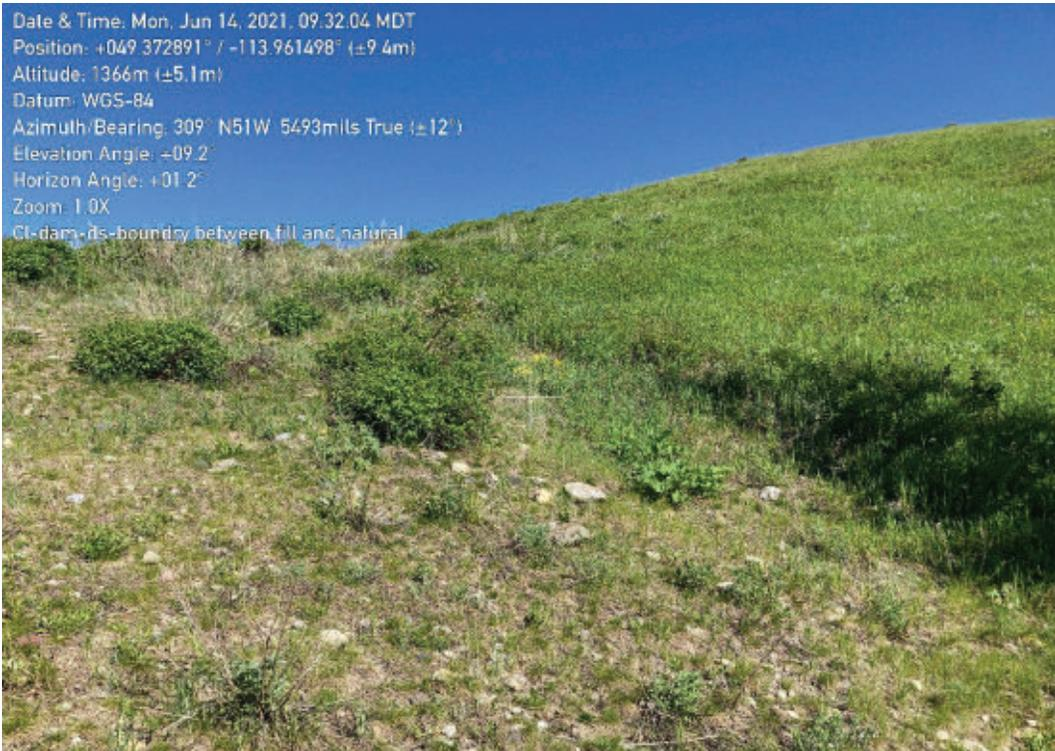
Photograph 1-14 Possible boundary between fill and natural materials, where different vegetation growth can be observed along the north edge of the downstream slope
