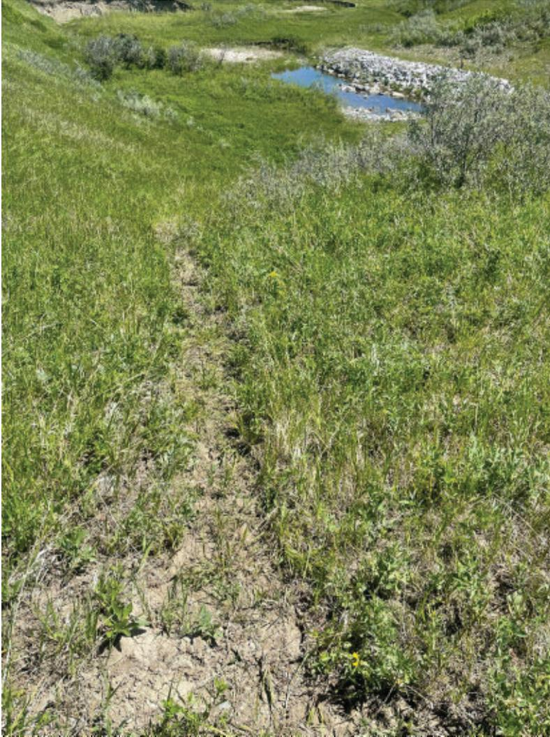
Photograph 2-17 A minor erosion or trail was observed along the north edge of the downstream slope at the abutment interface, looking down from the crest
