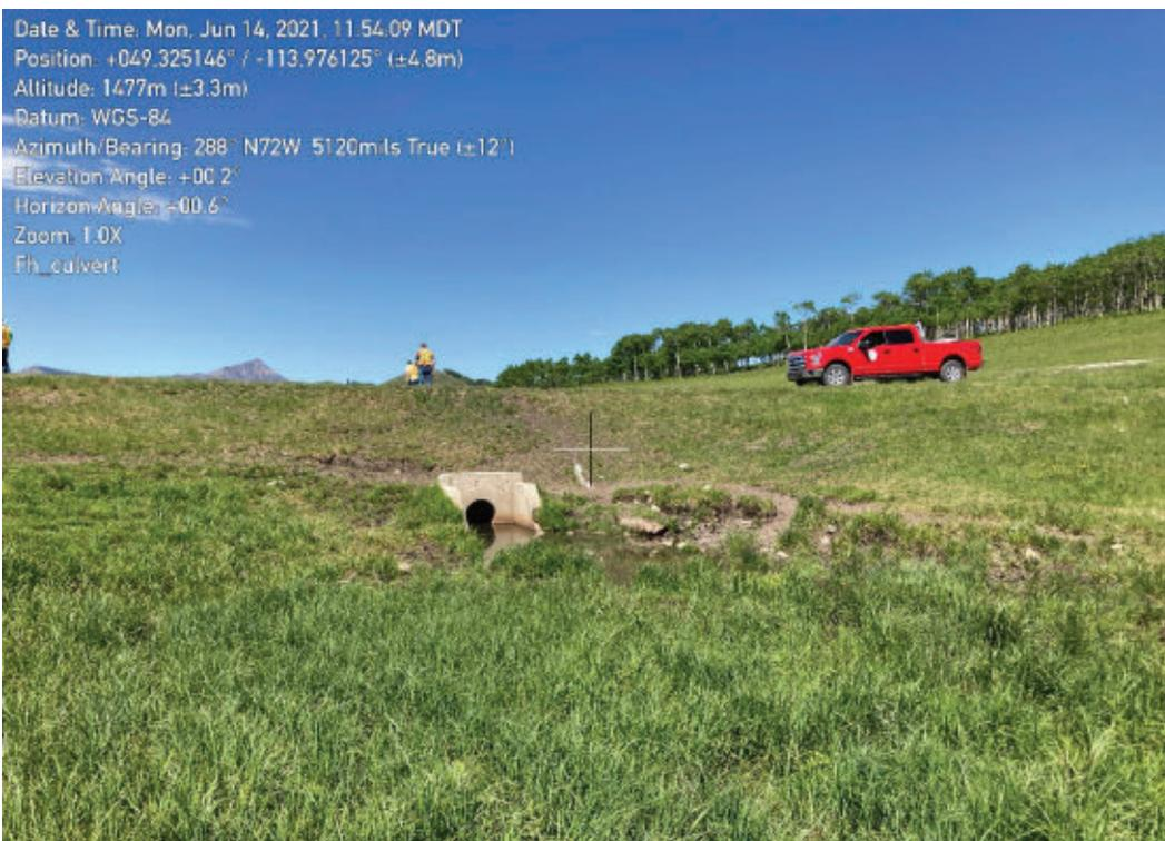
Photograph 5-10 Low level outlet headwall and outlet CSP culvert
