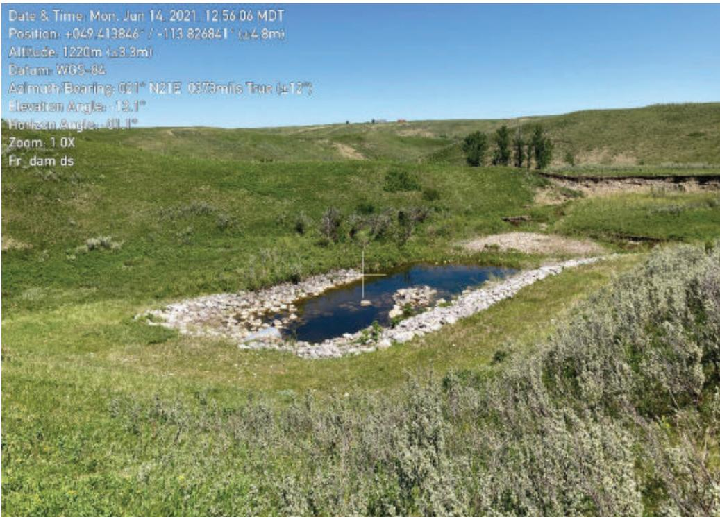
Photograph 2-8 Low Level Outlet CSP pipe and riprap at downstream toe, looking down from the crest
